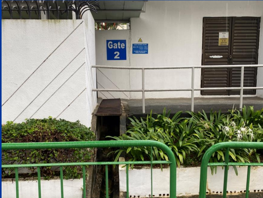
Side Gate 2 beside main entrance
